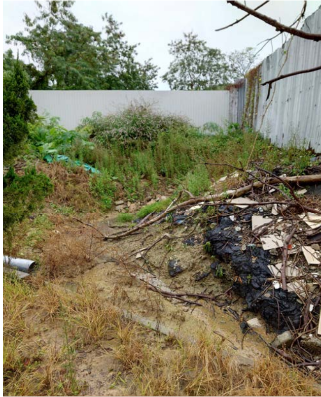
Photo View - P1 (Existing streamcourse blocked by other lot owner)
